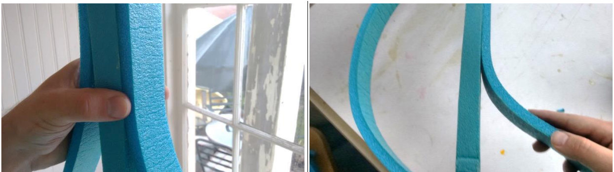
Figure 4.9 Placing the Layer
