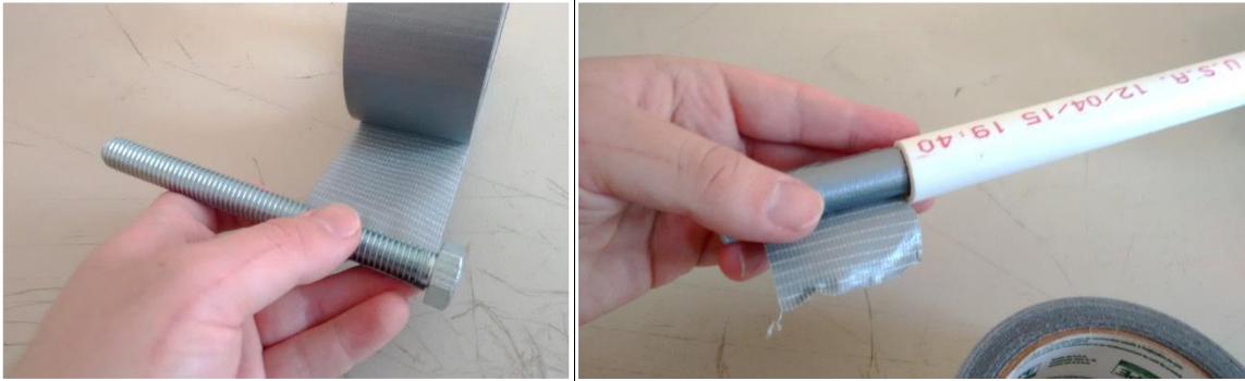
Figure 5.1 Sizing the Bolt
